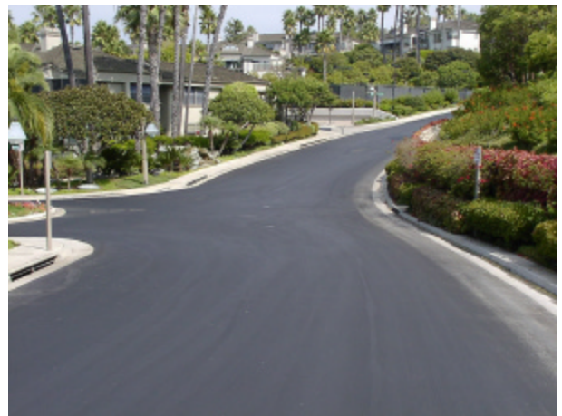
Notice there is only staining on the water side.
